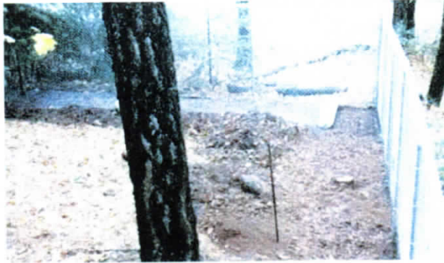
2' – 4' of fabric laid on the ground to prevent the burrowing of feral hogs. Ground cover to be likely raked back and then re-applied over the fabric.
